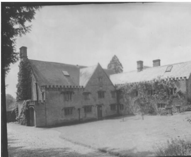
East - west range of Williamscot House east-west range
