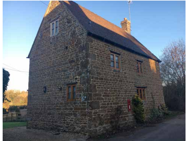
Post Box Cottage
