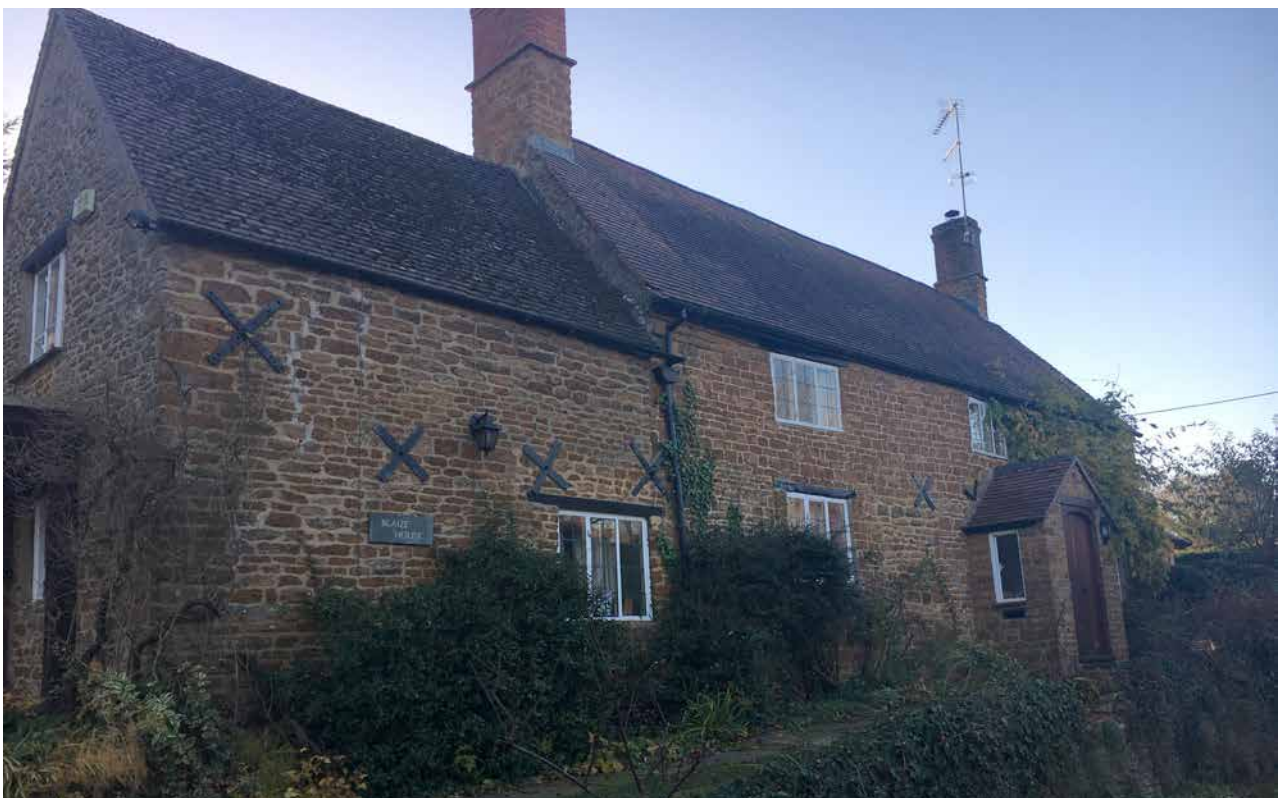
Blaize Farmhouse (former Public House)
